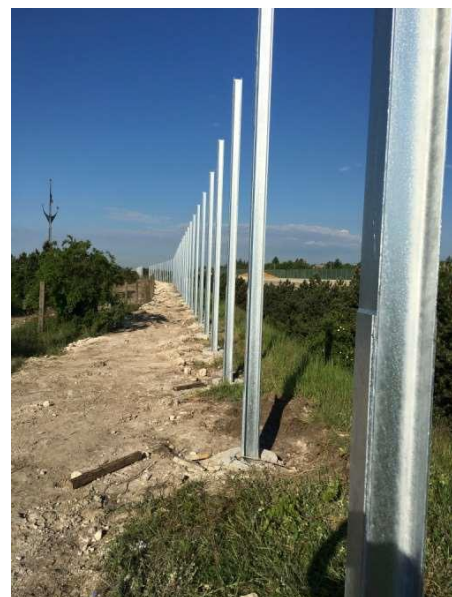
Post setting – can be seen clearly on the belts used reinforcements
