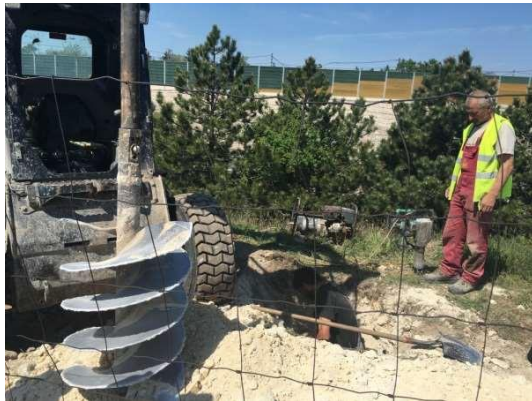
Base structure drilling
