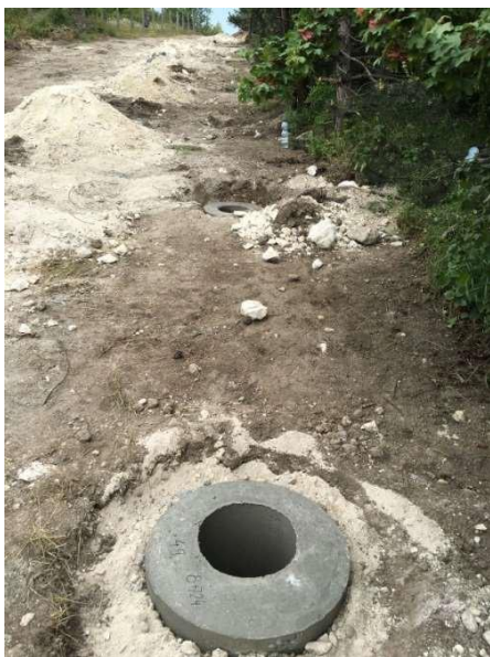
Concrete base structure, with a cup formed for the post
