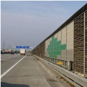
PIN on the noise barrier
