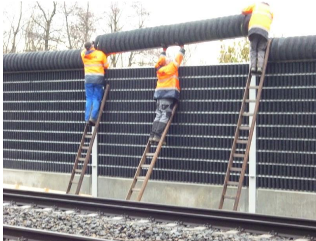
Manual installation of A PIN A Lärmspoiler® next to railway traffic, without track obstruction
