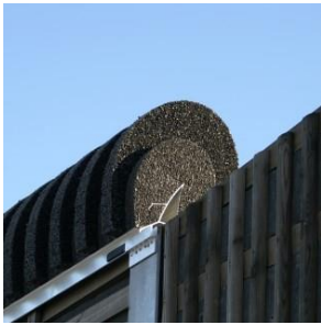
Installation on the posts
